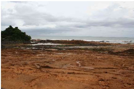
Figure 17. Near Lolabé a broad coastal strip of rainforest was seen cleared over several km (a sign indicated involvement by 'Razel' a French company), reportedly for construction of roads and a deep-water sea port.
