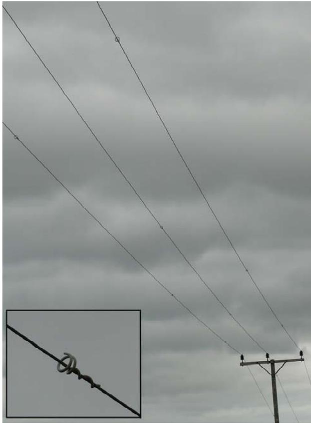
*Figure 19. Medium voltage distribution line with small spirals (so-called 'pig tails') placed at regular intervals in the conductors as bird flight diverters (Photo: Bureau Waardenburg).*
