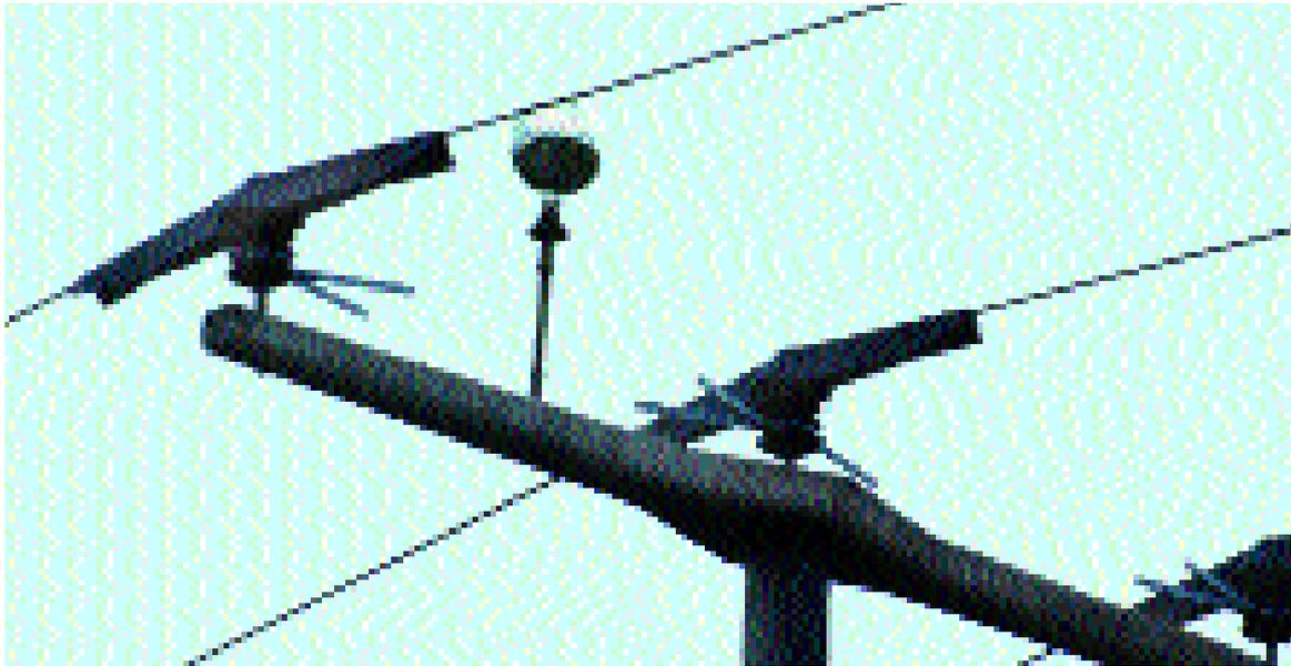
*In the past reflecting glass balls were used first on this pole and were later replaced by bird diverters. It was not until in a third attempt that the insulators were effectively covered with molded plastic hoods.*
