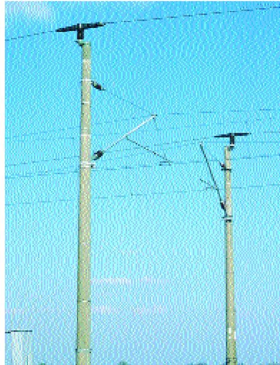
*A favorite perch site but dangerous as well: the pole top of transmission lines of the German Railway Company. The energized power line is attached to the pole top. To reduce the shock hazard the power line was covered with insulator hoods 130 cm in length later on.*
