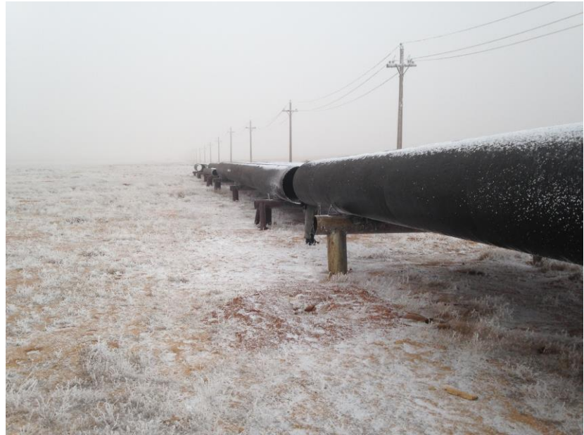
Pipelines can be significant barriers to large mammal movements. However, placement of pipelines underground can often solve this problem. ©WCS/K.Murphy
